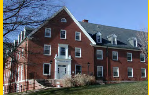
Dorchester Hall Renovation (2018)
